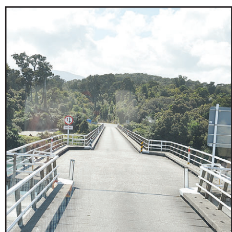
One lane bridges like this are a common sight in New Zealand. The wide area in the center is to provide room for approaching vehicles to pass one another.
